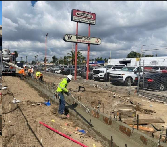
09/16/2024: Concrete Pour along Segment 2C for Curb & Gutter.
