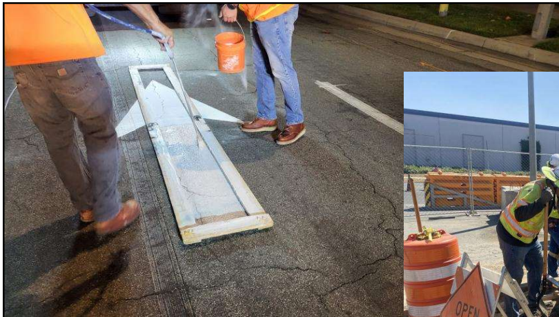
09/09/2024: Painting and Glass Beads for the Type 1 Arrows in Segment 2A & 2B.
