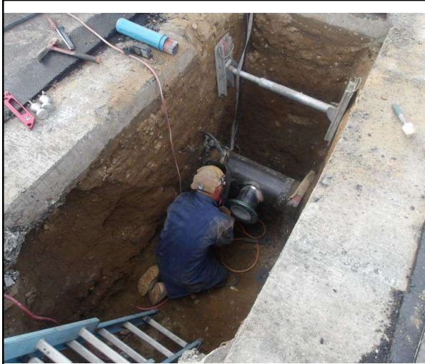
09/18/2024: Griffith Crew Installing 6" Gate Valves to FH Main Set for Tapping
