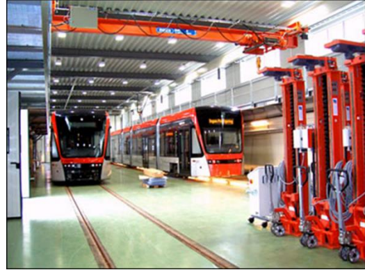
Figure 3-4: Overhead Crane and Heavy Maintenance Area
