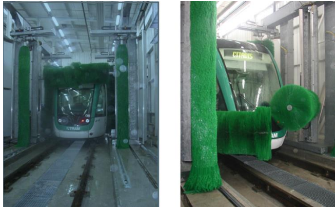
Figure 3-2: Drive Through Wash Plant
