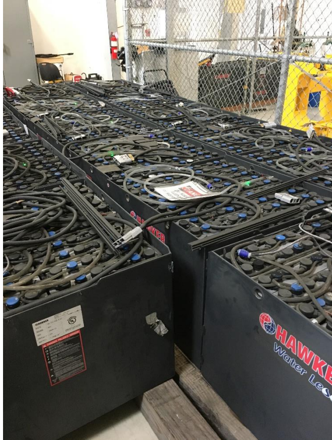
Figure 4-10: Battery storage area at Long Beach Container Terminal
