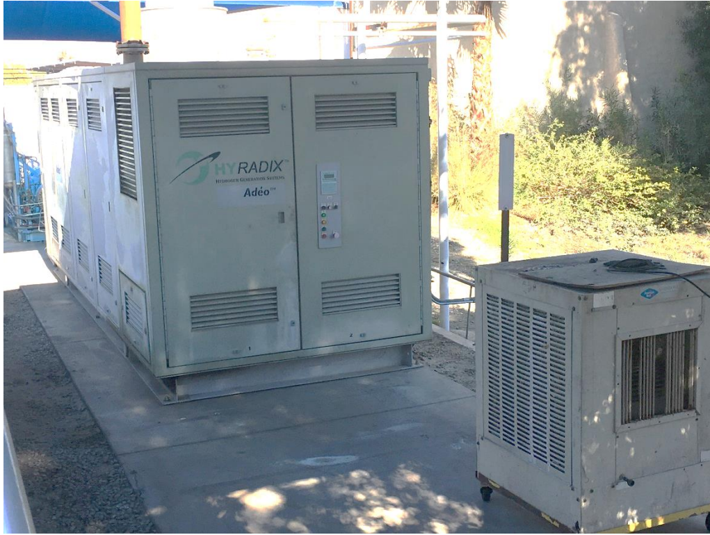
Figure 5-7: Typical hydrogen production facility
