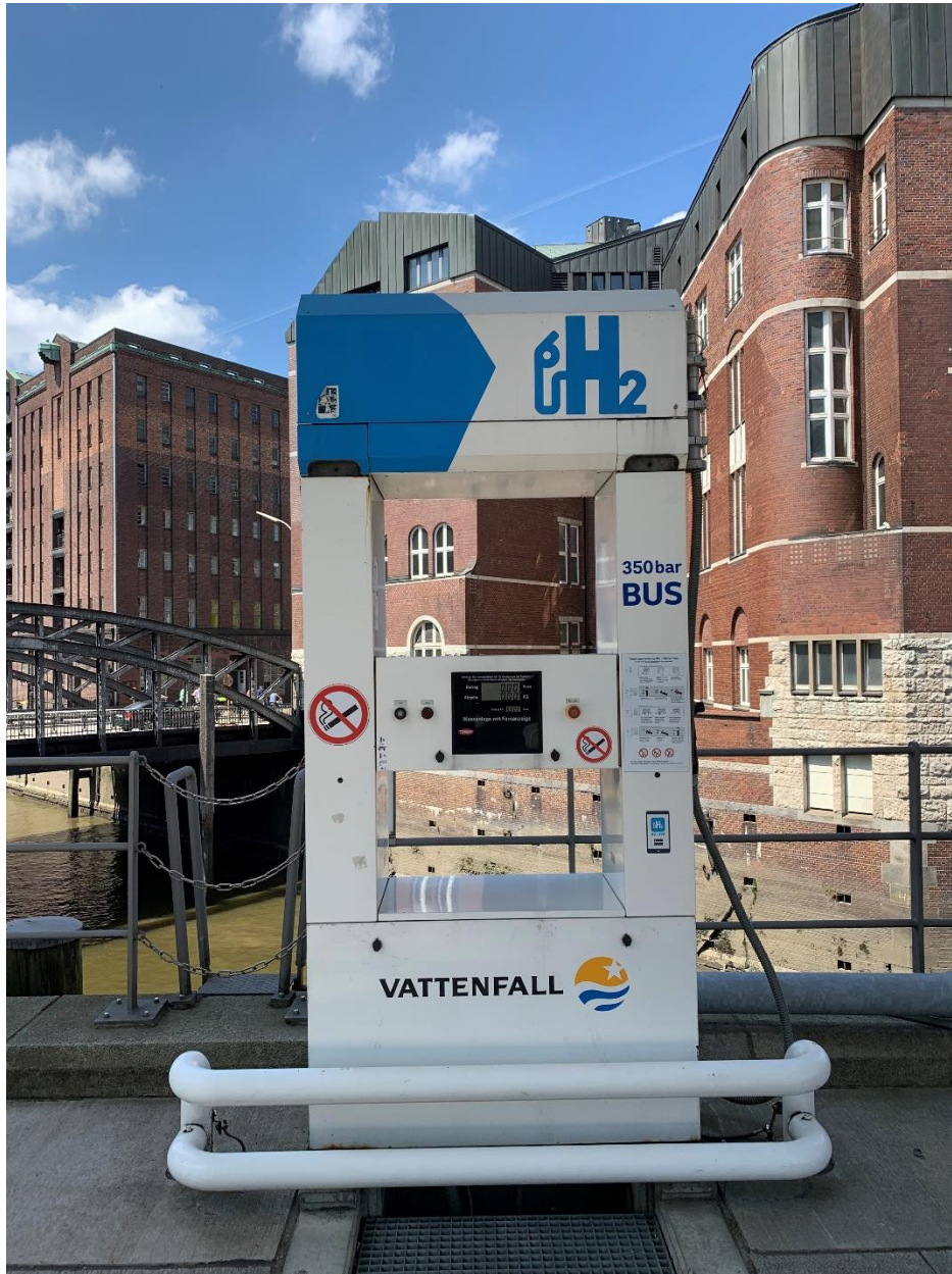
Figure 6-6: Permanent Hydrogen Refuelling Dispenser (Hoffrichter, 2019)
