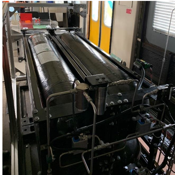
Figure 2-16: 350bar Hydrogen Tanks Installed on a Train
