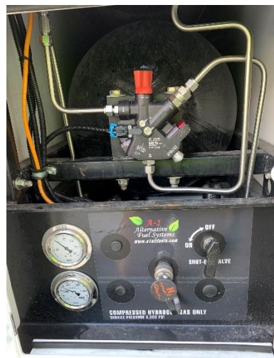
Figure 2-15: 350bar Hydrogen Tank Installed in a Truck (Hoffrichter, 2019)
