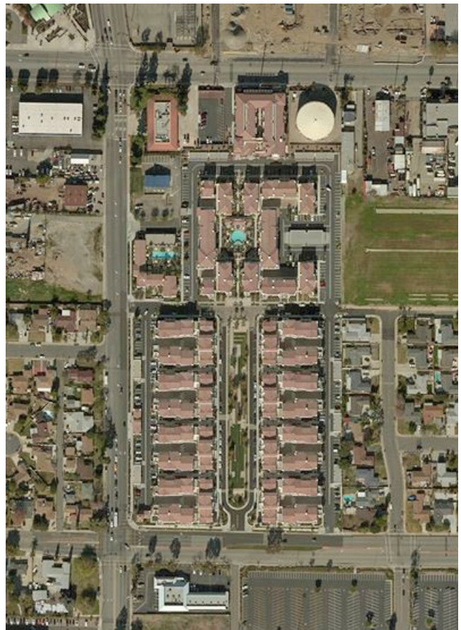
AERIAL PHOTO OF THE PASEOS IN NORTH MONTCLAIR
