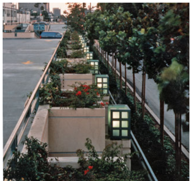
PARKING STRUCTURE IN SANTA MONICA, CA
