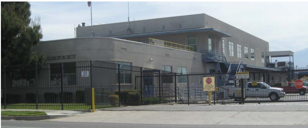
Photo 4.6-6. Southern California Gas Company North Building
