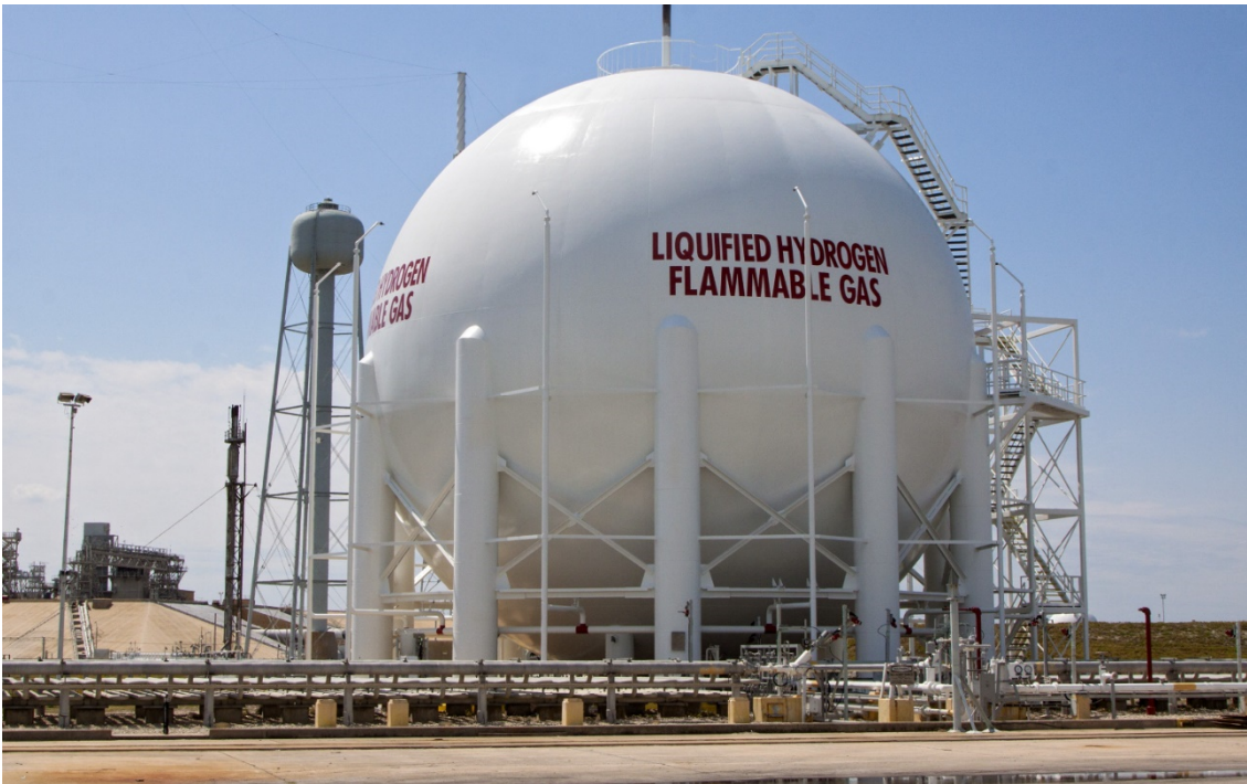
Figure 16. Newly Refurbished Liquid Hydrogen Storage Tank at Launch Pad 39B at NASA's Kennedy Space Center
