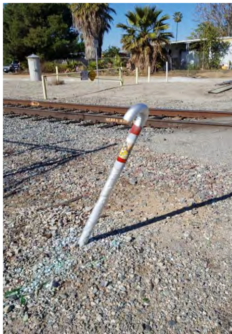
Photograph 12: Unmarked breather pipe (one of four) at SFR ROW and South Eucalyptus Avenue.
