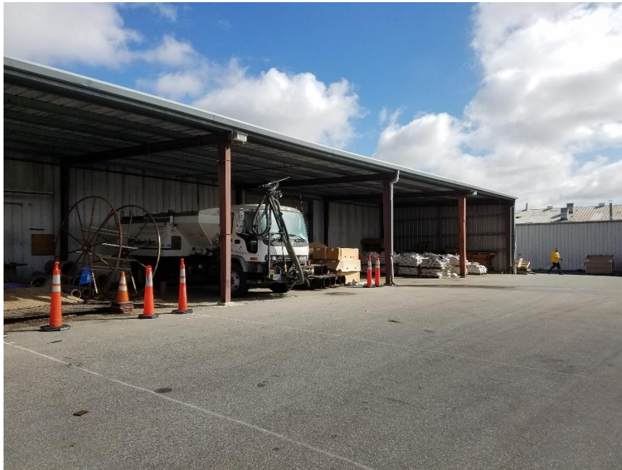
1. View looking northeast at Warehouse 2 located at 1333 S Bon View Ave.
