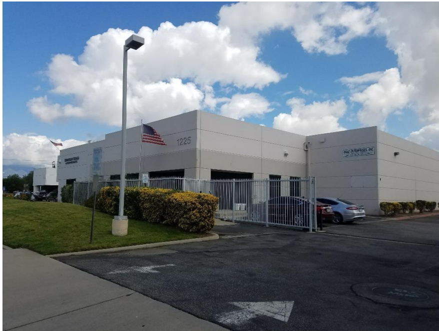
7. View looking north at adjacent building located at 1225 S Bon View Ave.
