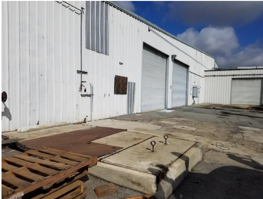
3. View looking in Warehouse 2 on east side of warehouse, at a capped water well
