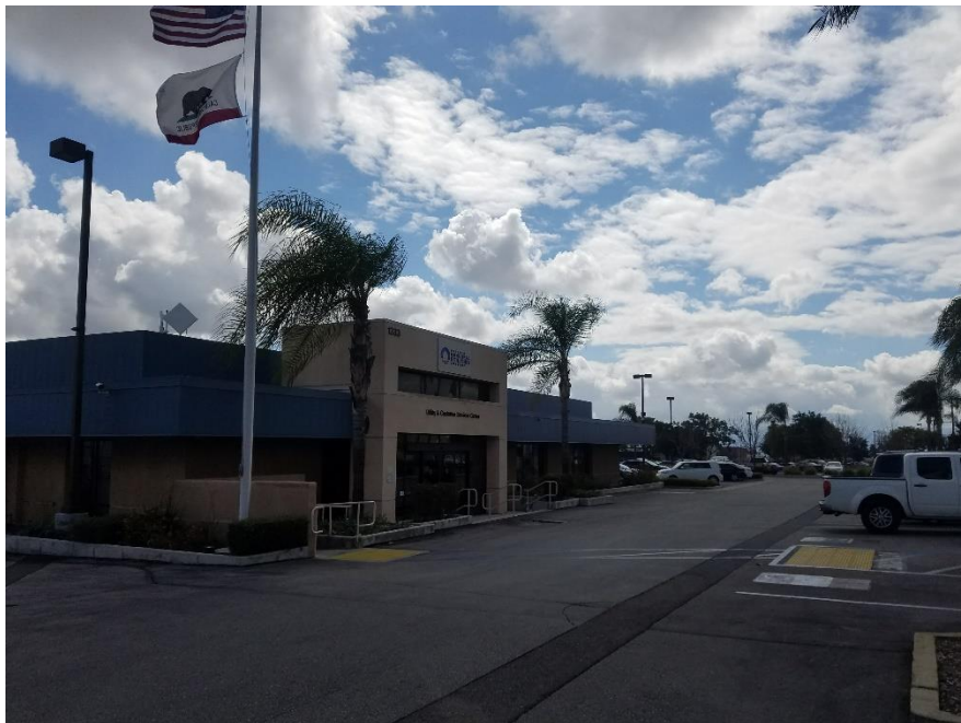
8. View looking southeast at Site at main office located at 1333 S Bon View Ave.
