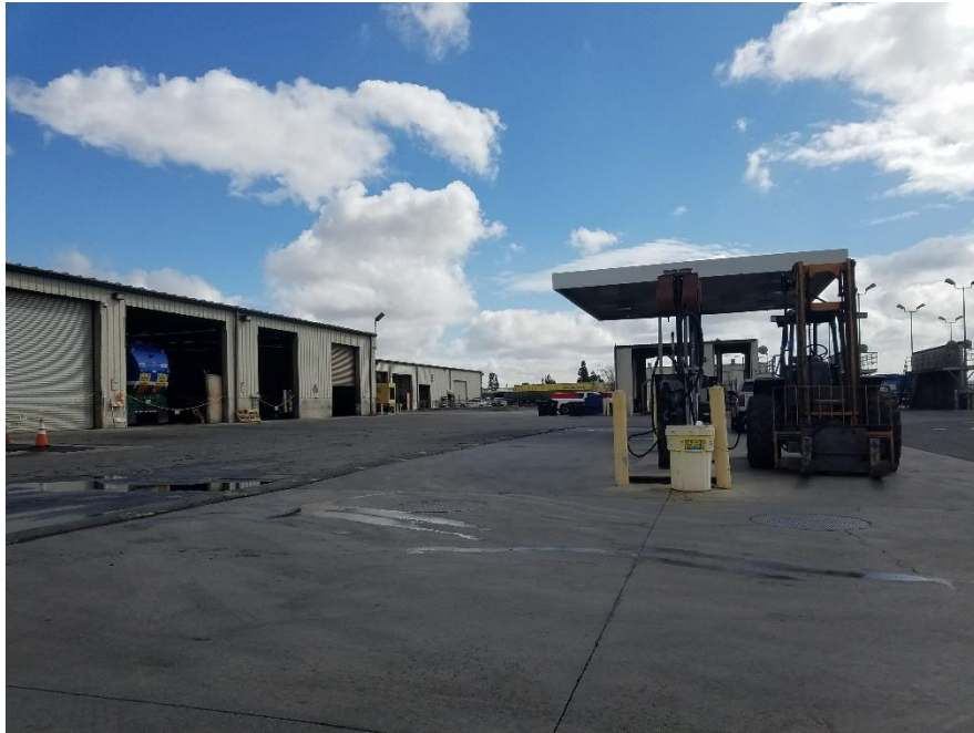
9. View looking east at the CNG station located at 1425 S Cucamonga Ave.
