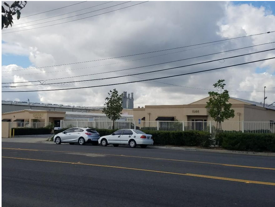
6. View looking west at adjacent building located at 1344 S Bon View Ave
