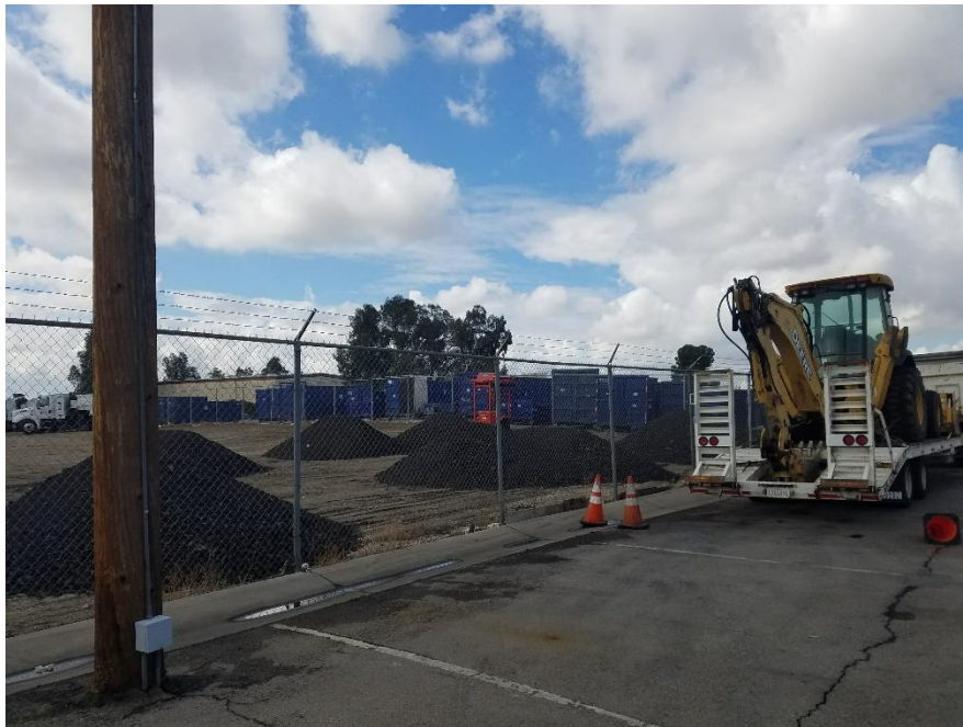
6. View looking south at 1516 S Cucamonga Ave
