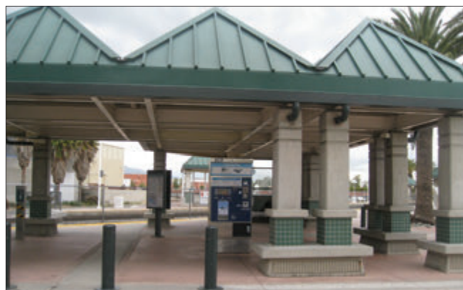
EXISTING CONDITIONS OF AMENITIES AT THE METROLINK STATION AND ITS CONTEXTUAL RELATIONSHIPS
