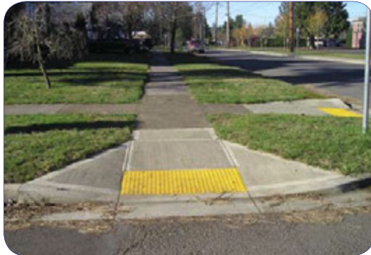
Curb ramps should be installed at each crossing approach.
