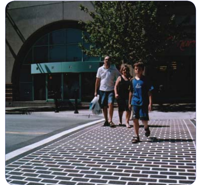
ThermoPrint or Duratherm are special thermoplastic products that produce highly reflective patterns
