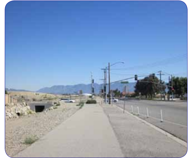
Existing Class I Bike Path is overgrown and unattractive to users.
