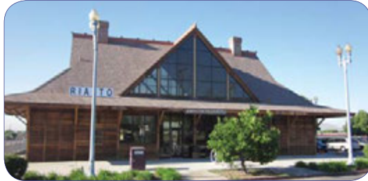
View of Rialto Metrolink Station
