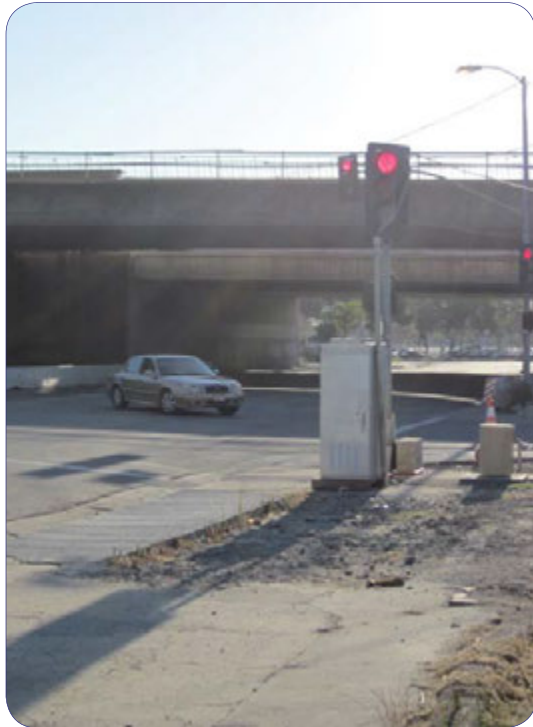
Construction hinders walking and biking connections to Carousel Mall
