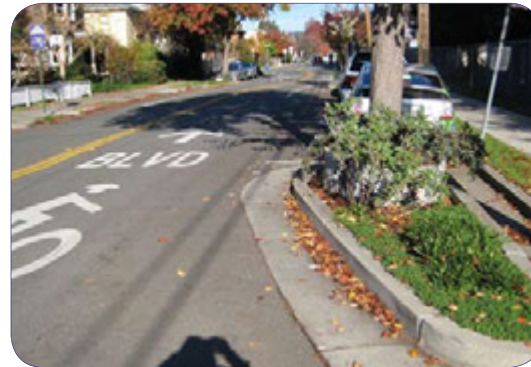
Chokers can reduce vehicle speeds by visually narrowing the roadway and requiring vehicles to shift their positions horizontally.
