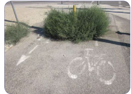
Unmaintained facilities discourage use and create hazards
