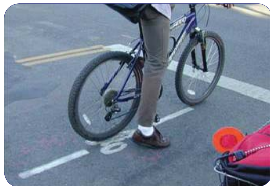
Bicycle detection at signalized intersections can be managed using bicycle loop detectors.
