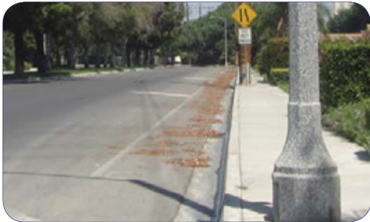
Unmaintained bike lane and non-ADA compliant sidewalk
