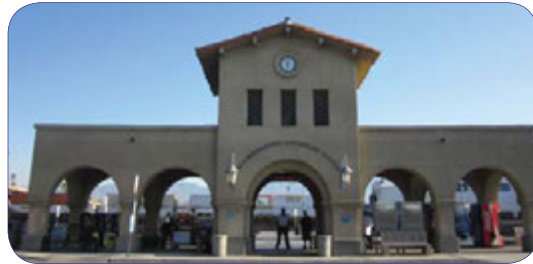
View of San Bernardino Metrolink Station
