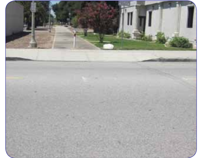
Along the Pacific Electric Trail, cities have often not improved mid-block crossings. This example is in Upland.
