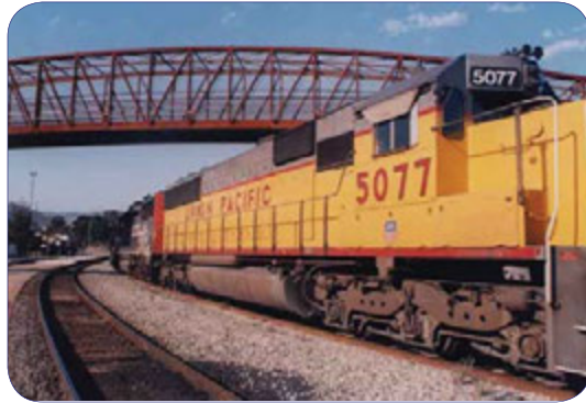
Overcrossings can provide access over railroad tracks for a more direct path of travel.
