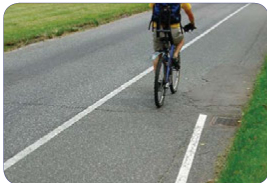
Sewer grates should be clearly marked so that bicyclists have time to avoid them.
