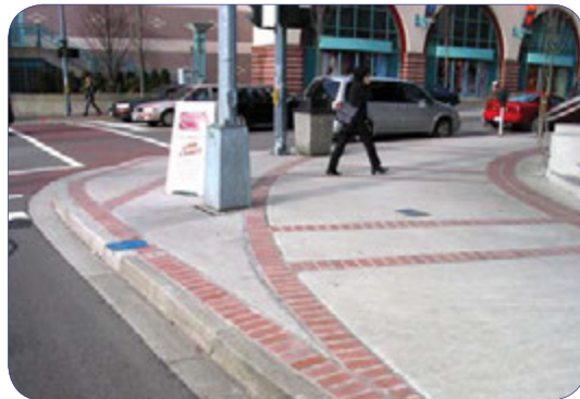
Reducing the curb radius at intersections causes motorists to lower speeds when initiating a turn.
