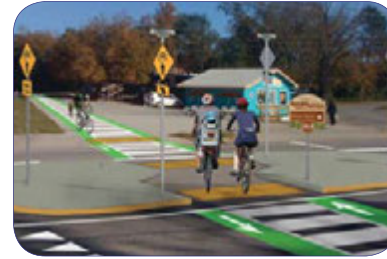
Pacific Electric Trail crossings should be high visibility, with marked crosswalks, signs, and yield pavement markings to improve safety for trail users.
