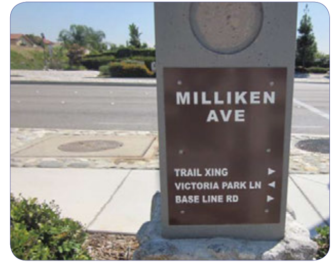
Existing wayfinding monument along Pacific Electric Trail.
