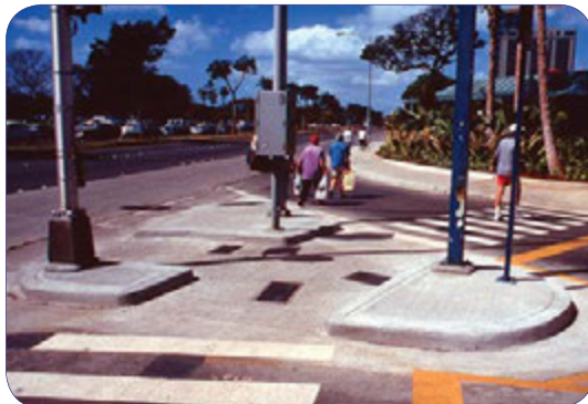
Triangular median islands allow pedestrians to cross right turn slip lanes and wait in the median until they have the right-of-way to cross.
