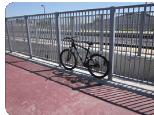
Illegal bicycle parking near tunnel to access Track 2.
