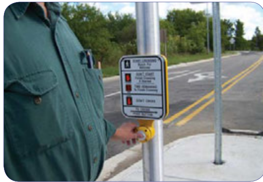
Pedestrian push buttons allow pedestrians to trigger the signal when motor vehicles are not present.
