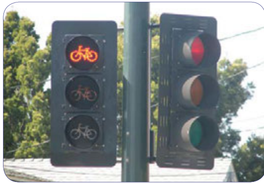
Bicycle signals provide a bicycle only signal phase for bicyclists to enter and exit bicycle facilities without conflicts with motor vehicles.
