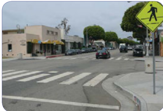
Advance stop bars should be installed with accompanying signage.
