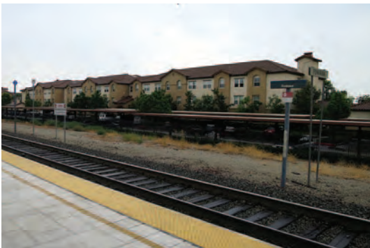
Fontana Station and adjacent housing.
