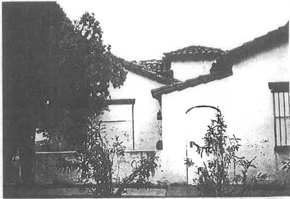
(Top) Detail of Roof lines and Fenestration at the Northeastern Corner of the Spanish Colonial Revival Style Residence.
