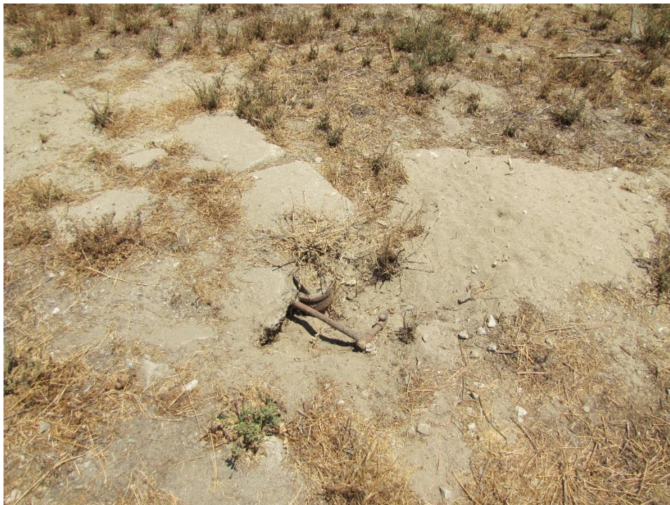
View of Utility Pipe within Concrete Foundation, 07/03/18
