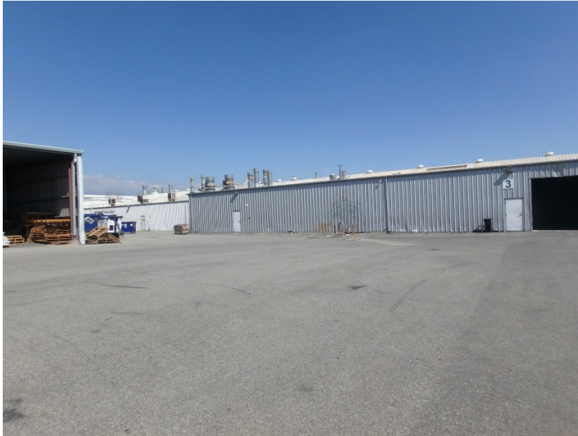
1533 S. Bon View Ave. View northeast of Building #2, showing original manufacturing shed portion from 1964 in center of photograph, with a later extension to its left (north). February 2018.
