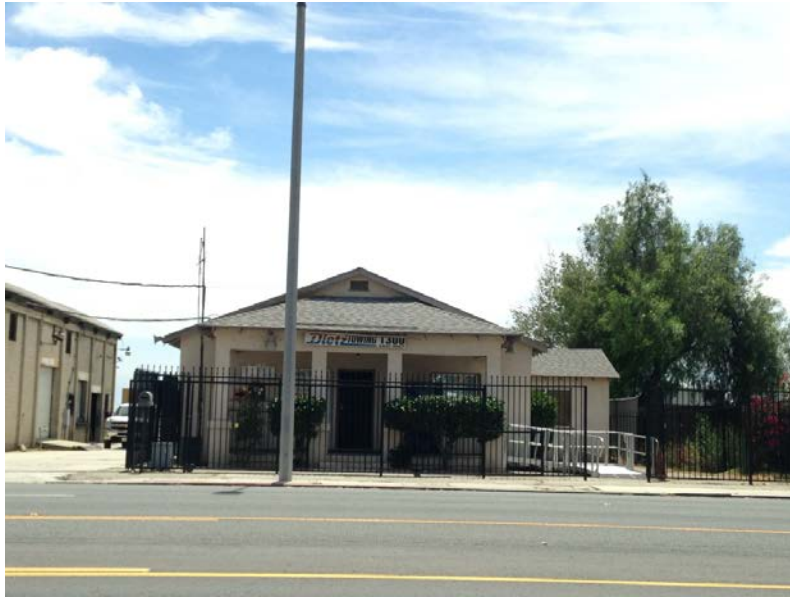
Building #2, former residence, front façade; view south
