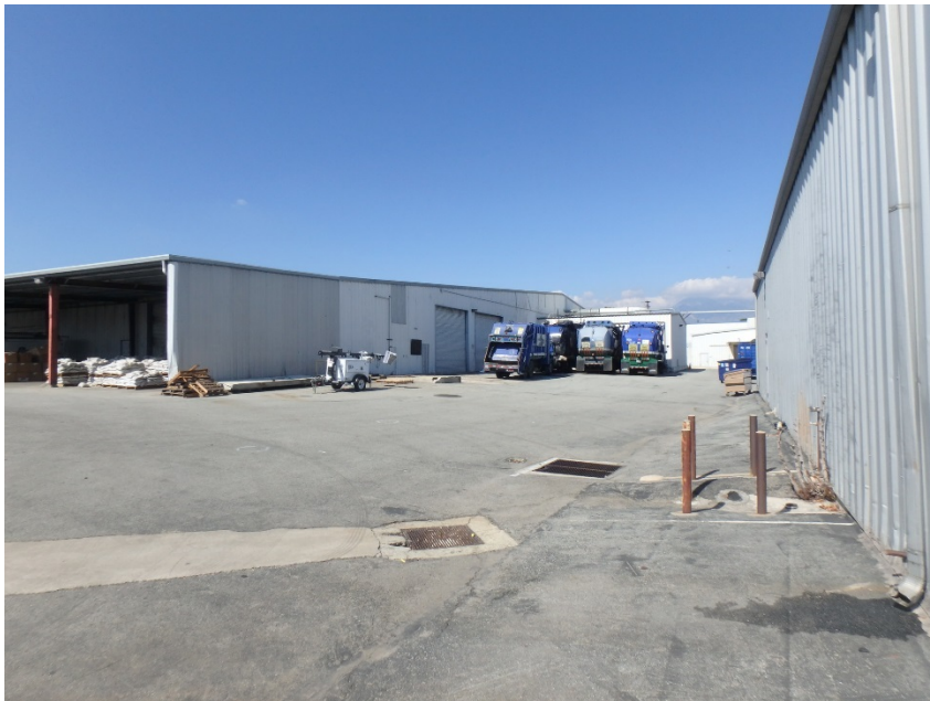
1533 S. Bon View Ave. View northwest Building #1. February 2018.
