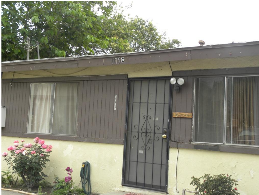
1175 Building 'C' E Holt. Blvd., June 2016
