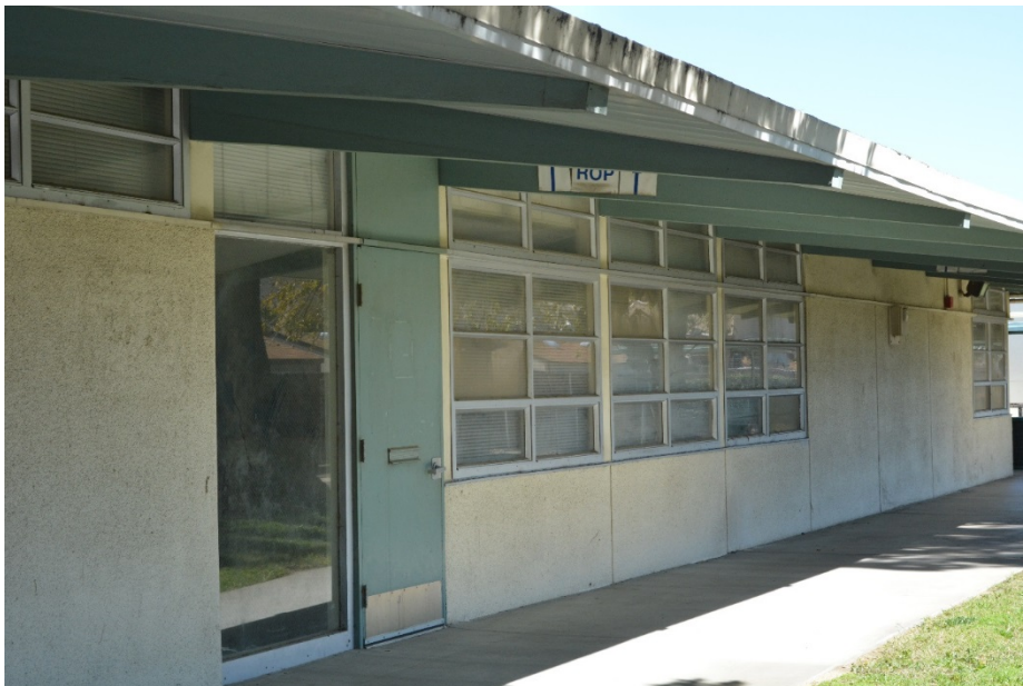
1501 S. Bon View Ave. Baldy View ROP. Detail of classroom window system and cantilevered roof eaves. South extent. March 2018.
