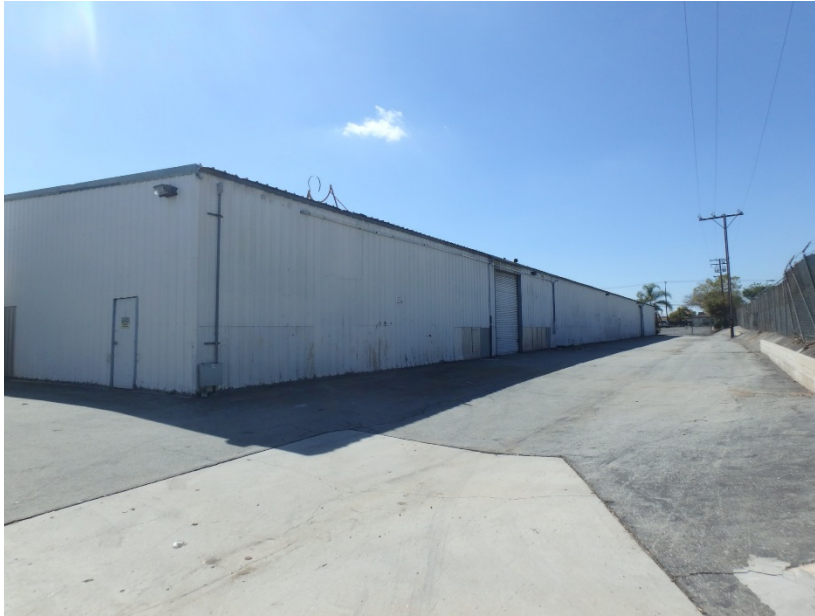
1533 S. Bon View Ave. View southwest Building #1. February 2018.
