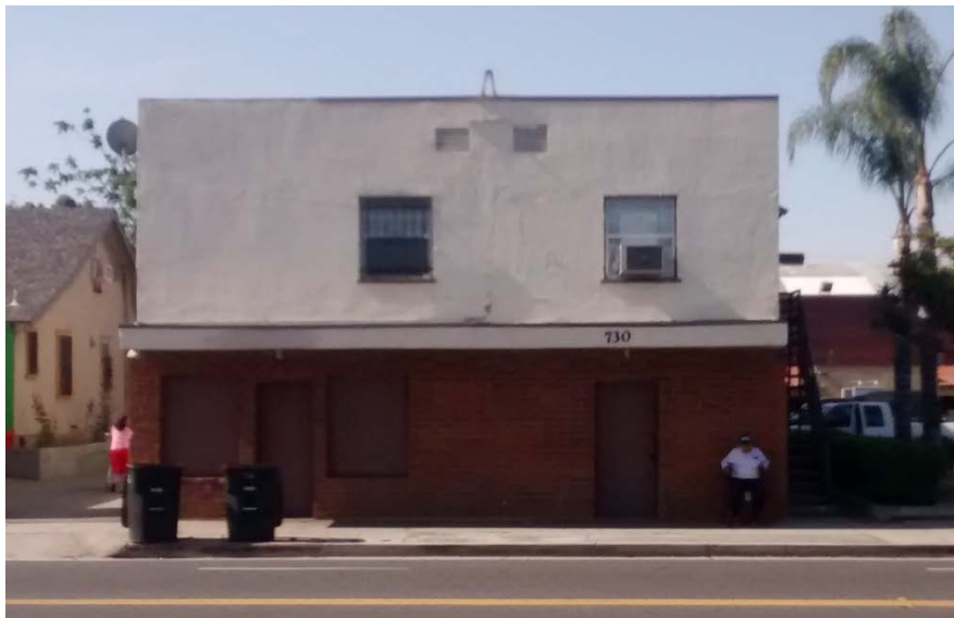
Former 730 E. Holt Blvd., Ontario; Facing South; 6/22/2016
