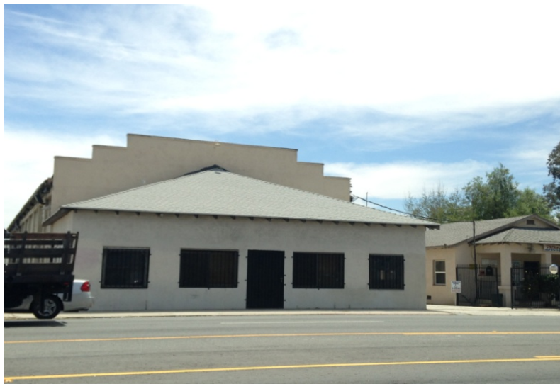
Building #1, former winery warehouse and store, front façade, view southwest
