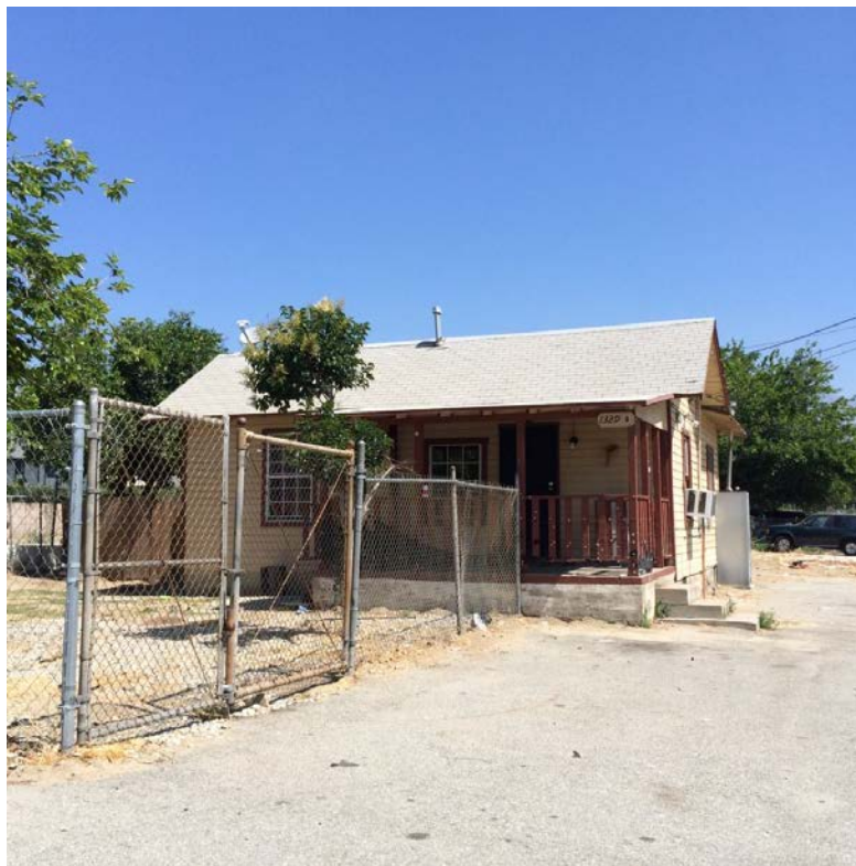
Facing North, June 2016
