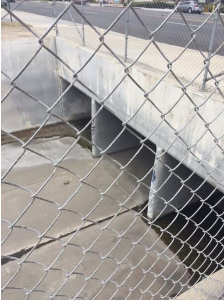
Photo 5. West Cucamonga Channel. The view is slightly northwest; photo taken June 13, 2016.
