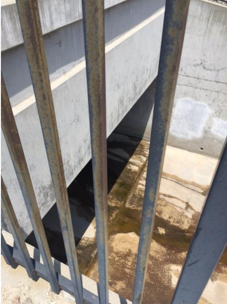
Photo 4. Day Creek Channel. The view is to the east; photo taken June 13, 2016.
