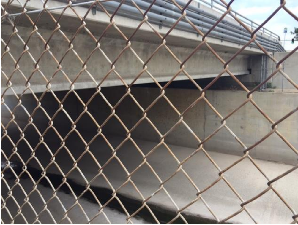
Photo 2. Cucamonga Channel. The view is to the east; photo taken June 13, 2016.
