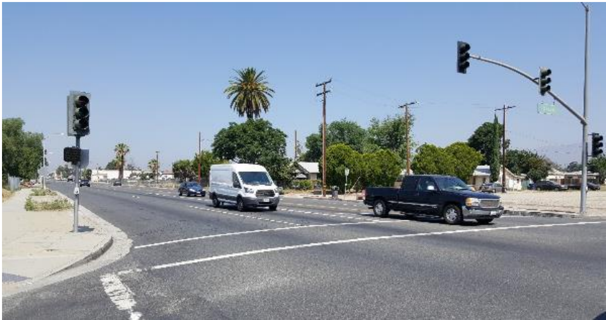
Figure 5-9: Existing Holt Boulevard at Grove Street, View Northwest
