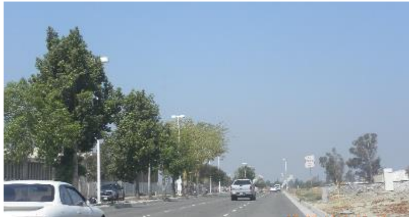
Figure 5-5: Airport Way, from the westbound lanes
