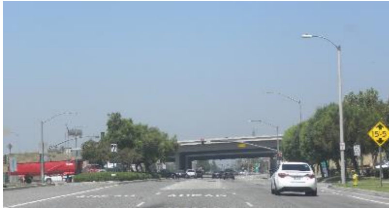
Figure 5-10: Foothill Boulevard at the Interstate 15 overcrossing, looking west
