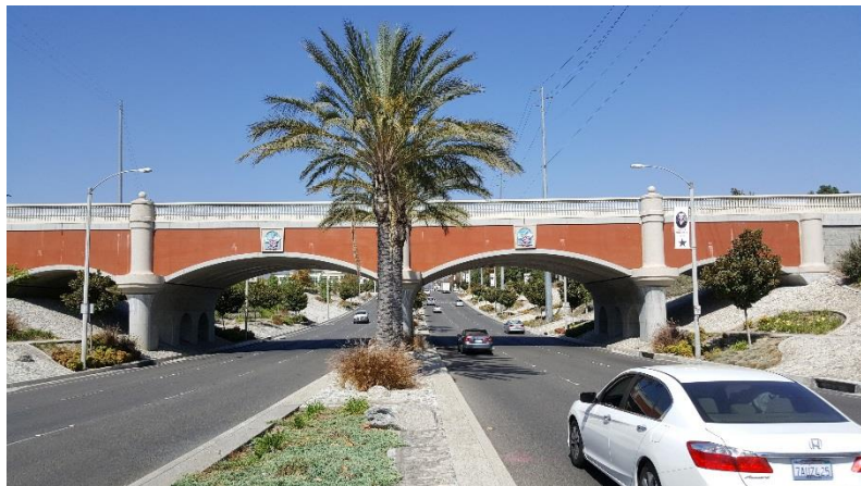
Figure 5-8: Haven Avenue at the Metrolink Railroad Bridge Crossing, looking north
