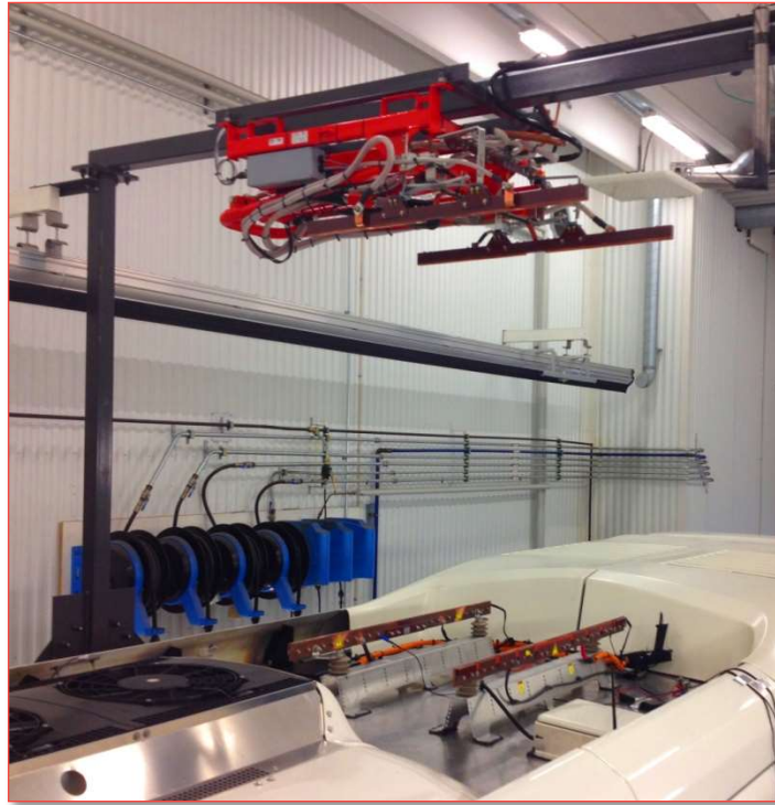
Figure 4-2. Inverted Pantograph and Charge Rails
