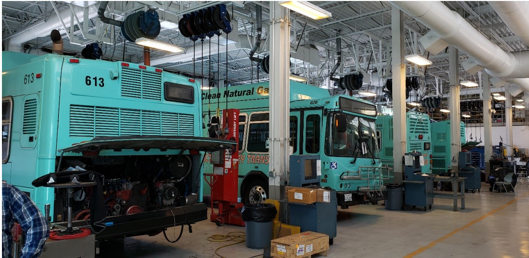
Figure 6-5. Hesperia Yard's Maintenance Bays
