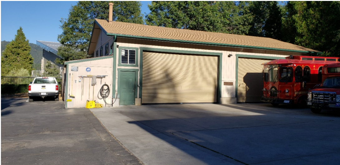
Figure 4-5. Crestline Base's Maintenance Facility
