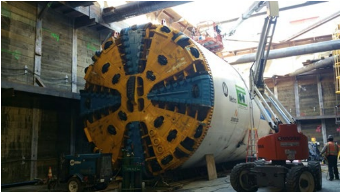
Figure 2: Tunnel Boring Machine
