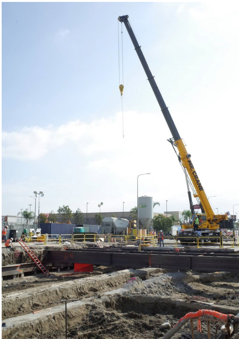
Figure 1: Example of Construction via Cut-and-Cover
