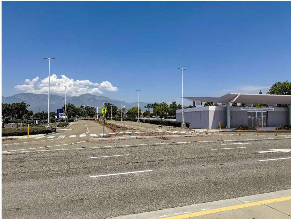
Figure 3.1-4 Visual Simulation View North Towards Terminal Way and East Way
