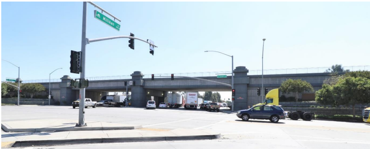
Figure 12: Southern Pacific Railroad Modern Grade Separation at Milliken Avenue and Guasti Road (View Southeast [9/30/22])
