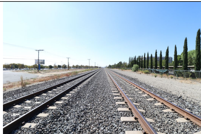
SPRR tracks taken facing west from a point approximately 1,100 feet west of Haven Avenue (9/30/22). Ontario International Airport is located to the south (left side of photo).
