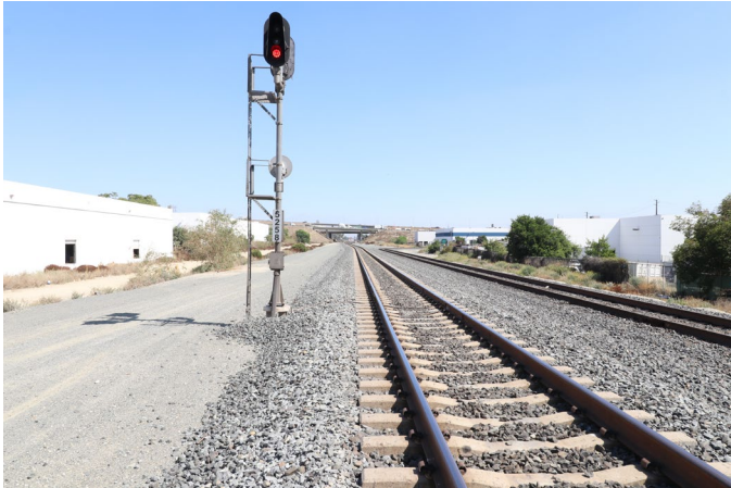
SPRR tracks looking east toward I-15 from a point approximately 1,900 feet east of Milliken Avenue, just east of the wall along the north side of the tracks (9/30/22).
