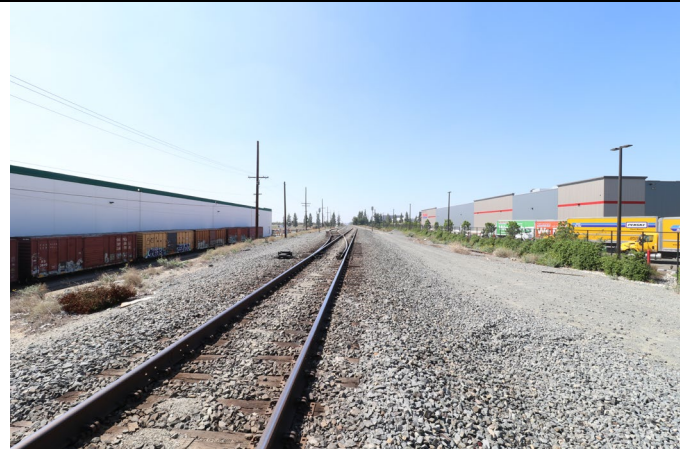
SPRR tracks looking west from the Guasti Road cul-de-sac (9/30/22).
