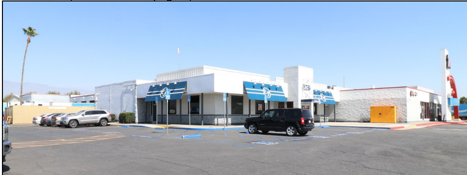
Commercial building, view northeast 9/30/22.
