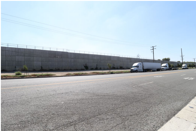
Wall associated with the modern grade separation along the north side of the SPRR tracks south of Guasti Road near Milliken Avenue. View southwest (9/30/22).
