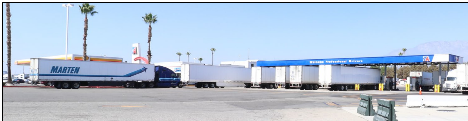
Overview showing fuel station canopies and a part of the commercial building, view northwest 9/30/22.
