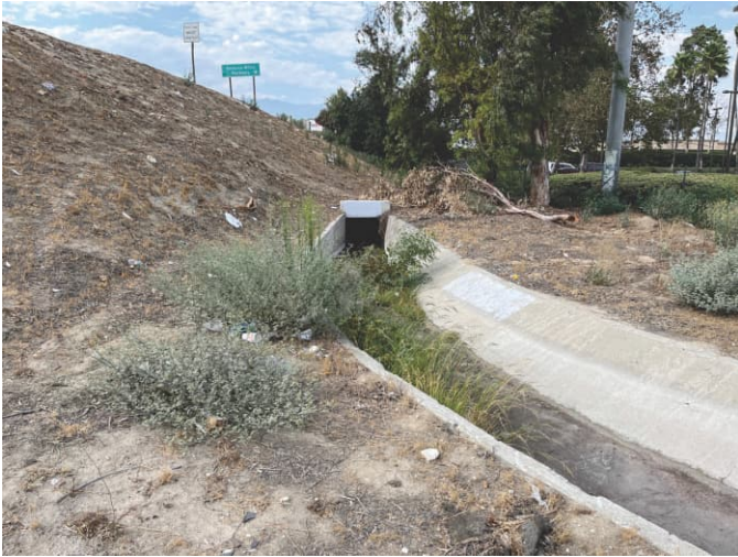
Photo 4: View of Feature 2, a concrete lined channel that is potentially jurisdictional.
