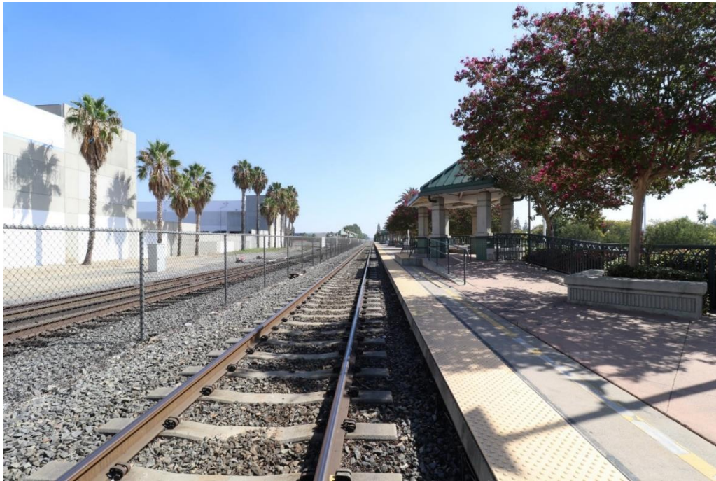
Figure 10: Atchison, Topeka and Santa Fe Segment (View East from the Western End of the Southern Metrolink Station Platform [9/30/22])
