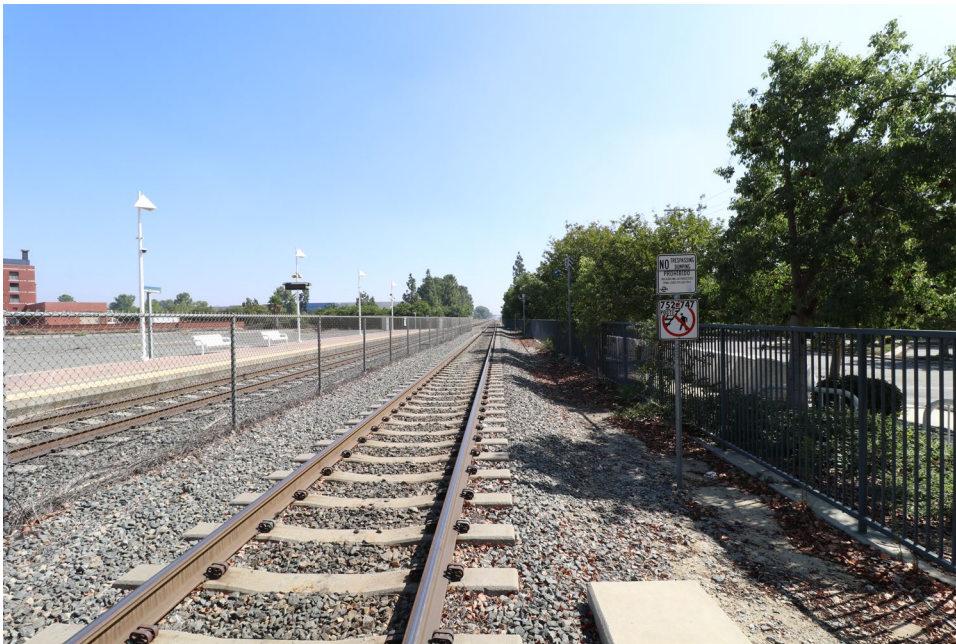
View east from the eastern end of the southern Metrolink Station platform (9/30/22).
