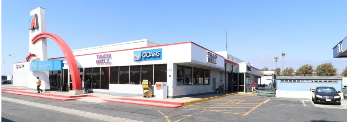
Figure 11: 4265 East Guasti Road (View Northwest [9/30/22])
