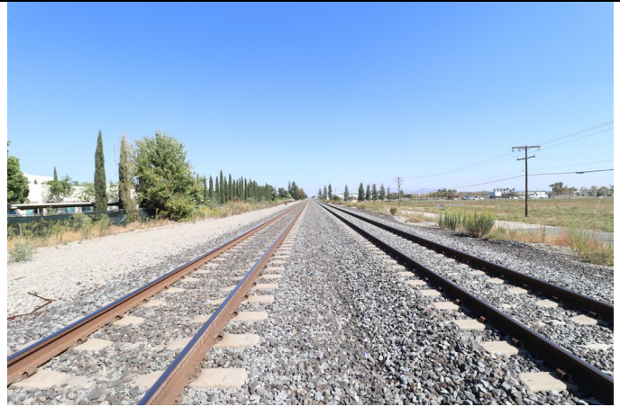
SPRR tracks taken facing east toward Haven Avenue from a point approximately 1,100 feet west of Haven Avenue (9/30/22).
