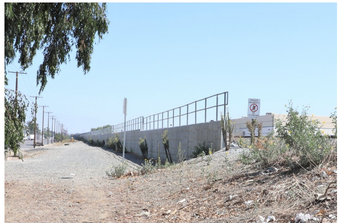
West end of wall associated with the modern grade separation on the north side of the SPRR tracks. Taken from the Guasti Road cul-de-sac approximately 500 feet west of N. Ponderosa Avenue. View east (9/30/22).
