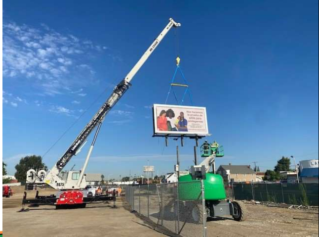
09/18/2024: Removal of Billboard at Sta. 448+78
