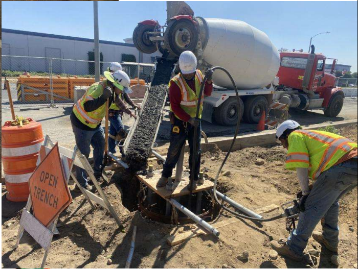
09/18/2024: Traffic Signal Foundation
