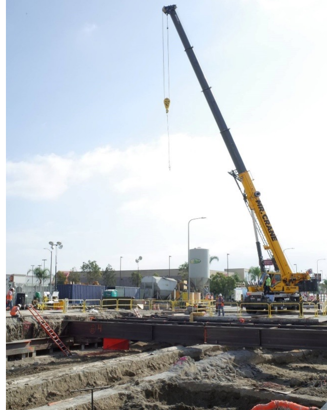
Example of Cut-and-Cover Construction
