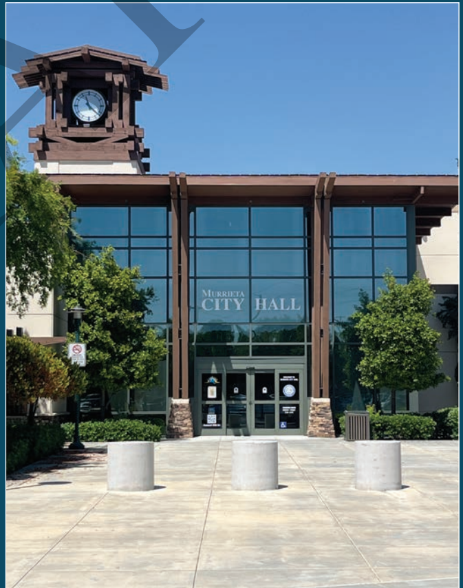
City of Murrieta City Hall
