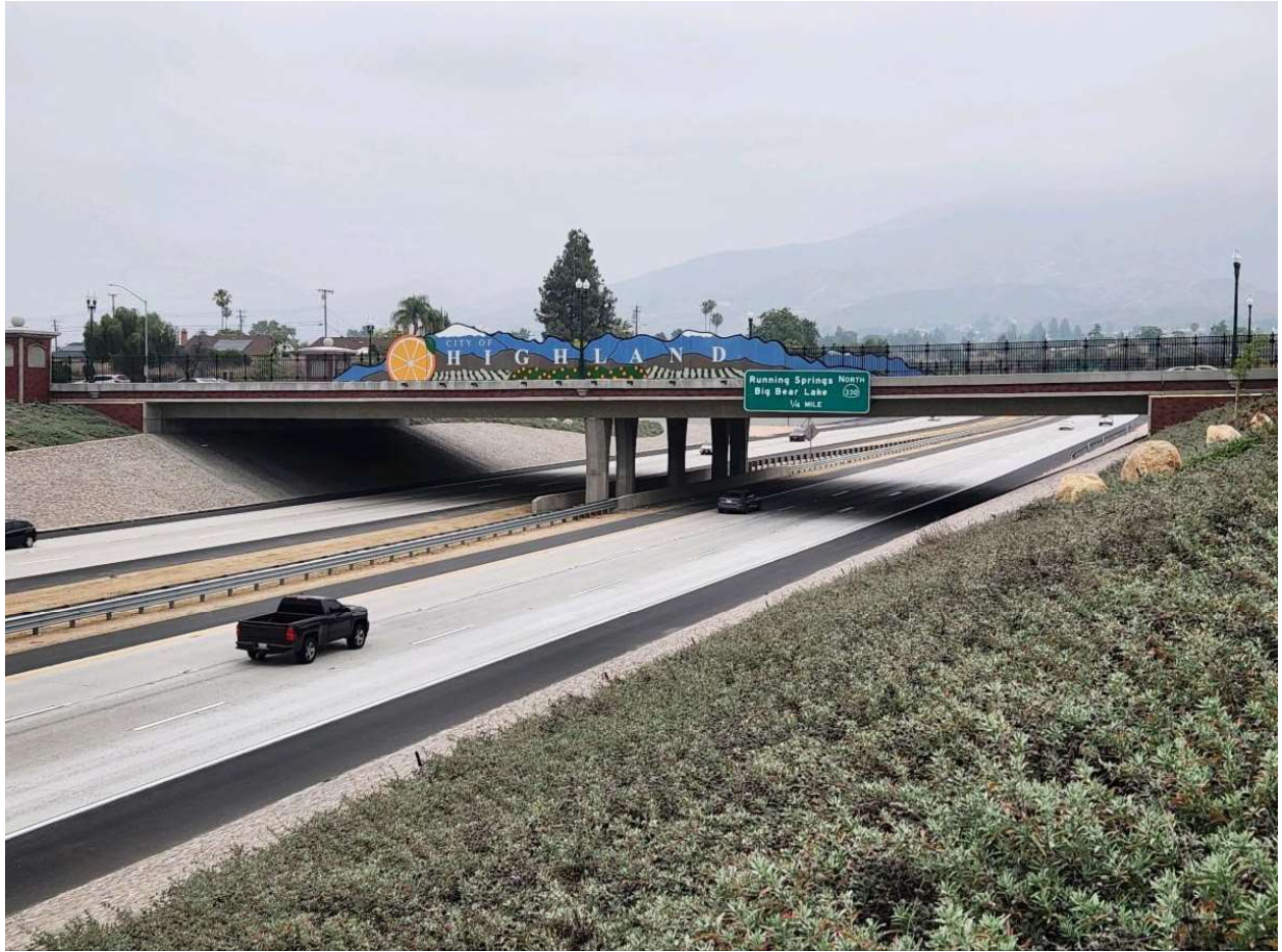
The City of Highland adorned the new bridge at Baseline at State Route 210 with a sign showcasing its pride as the gate way to the mountain communities. The bridge was reconstructed as part of the State Route 210 Lane Addition Project.
