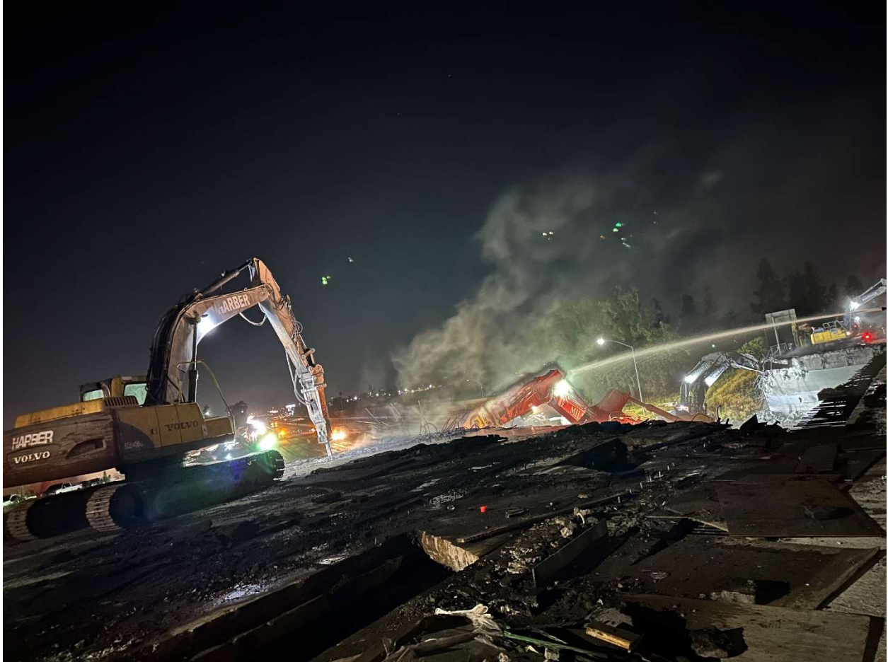
Nighttime work is necessary to minimize disruption to the traveling public. Crews are seen here demolishing the Vineyard Avenue bridge.
