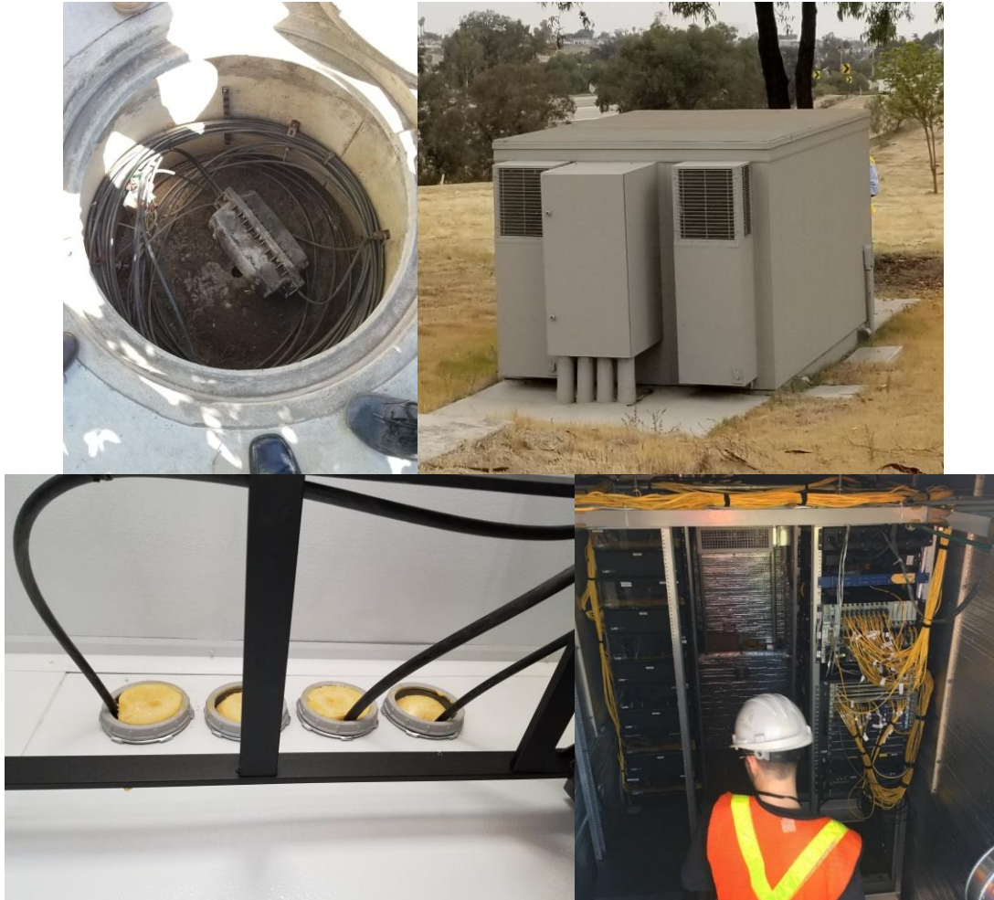
Figure 5-14: Typical Broadband Enhancement Node Connection
