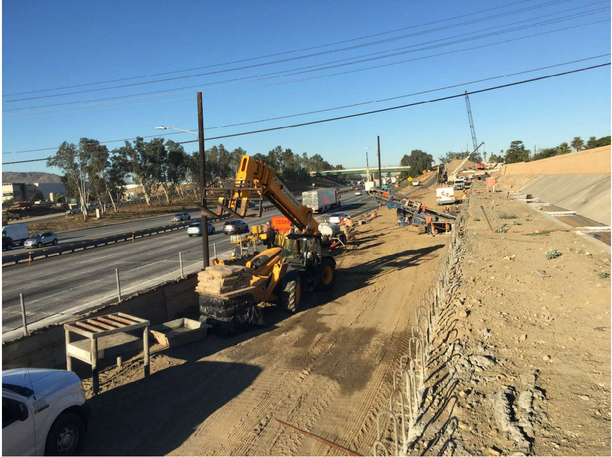
Preparing for the installation of new retaining walls along the ramps at Cedar Avenue in Bloomington, crews install the soil nail system for additional strength of the walls.
